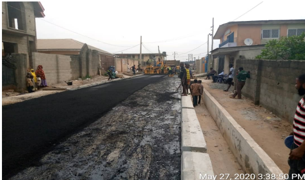
PRIMING, LAYING OF ASPHALTIC CONCRETE PAVEMENT
